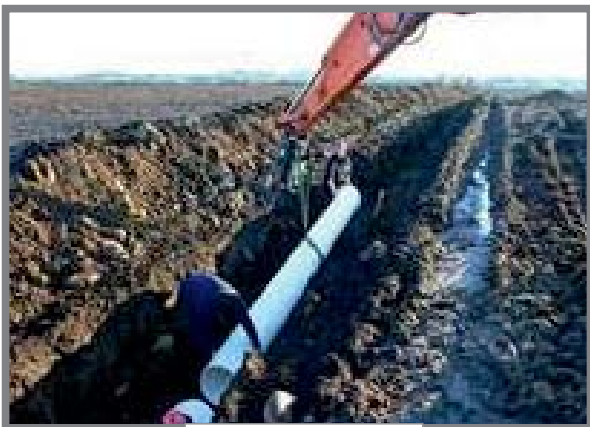
PVC pipe Installation
